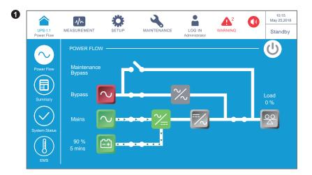
The screen above indicates that the UPS is in **Standby** mode. The inverter is off and the bypass input is out of the range.
